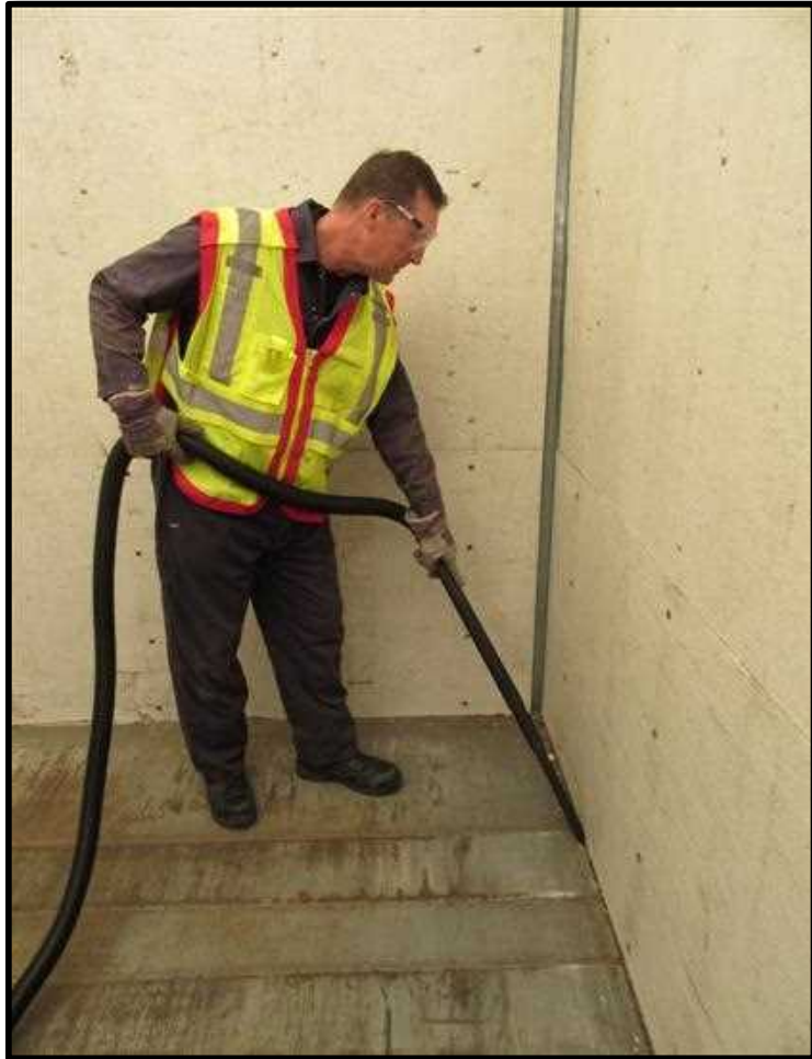
Eliminating Contaminants – Vacuum, Broom, Blower
